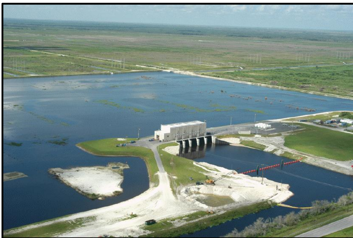
Figure 1-1 Aerial view of STA (Gonzalez, 2010)
